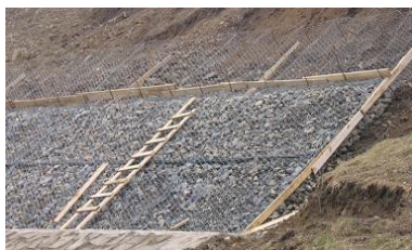
http://lt.lt.allconstructions.com/portal/categories/309/1/0/1/article/18712/gabionai-kas-tai-yra-ir-kur-naudingi pav. Pintos vielos tinklas šlaito sutvirtinimui
